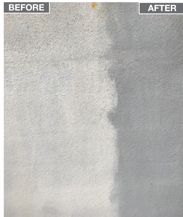
Oxidation on Stucco Left Side Before, Right Side after Being Cleaned with F9 BARC
