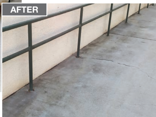
BARC Process #1 Rust from Metals Innovative Cleaning Services Phoenix, AZ
