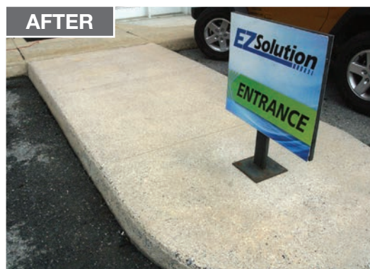
BARC Process #1 on Concrete Atkins Deck Treatment Service Inc. Leola, Pennsylvania
